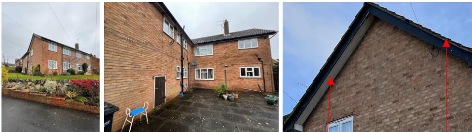
Laminated boards on the underside & fascia
