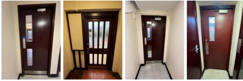
Communal doors with front and rear final exits doors with levered handles.
