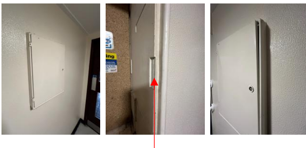
Damaged securing bead
