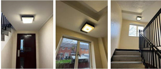
Communal area, stairwell emergency lighting
