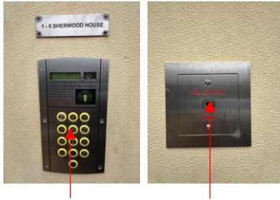
Intercom access and firefighter's switch
