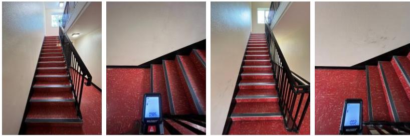
Ground to 1 st & 2 nd floor staircase.
