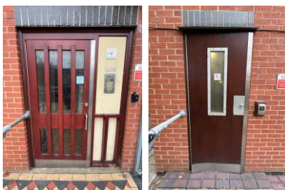
Front and rear entrances to block
