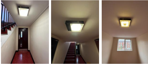
Communal area, stairwell emergency lights.
