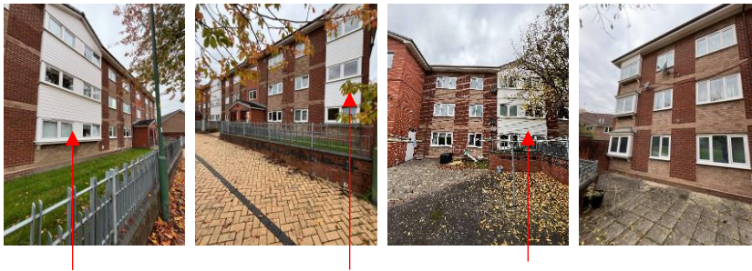
UPVC Shiplap cladding to the front and rear and UPVC window units
