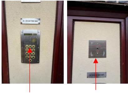
Intercom access and firefighter's switch
