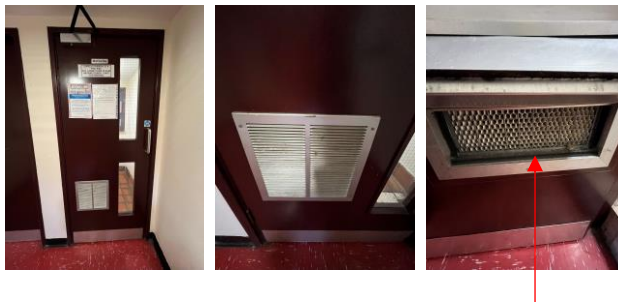
Refuse bin room door and ventilation intumescent seals.
