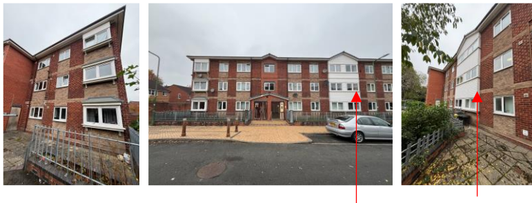
UPVC Shiplap cladding to the front and rear and UPVC window units
