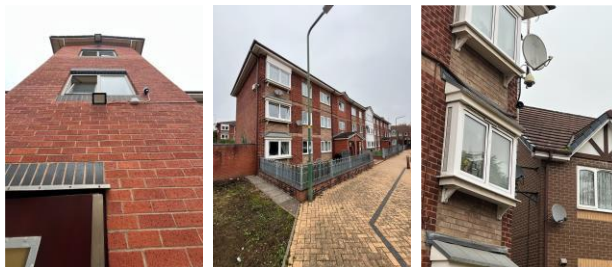
Rear lighting, & CCTV
