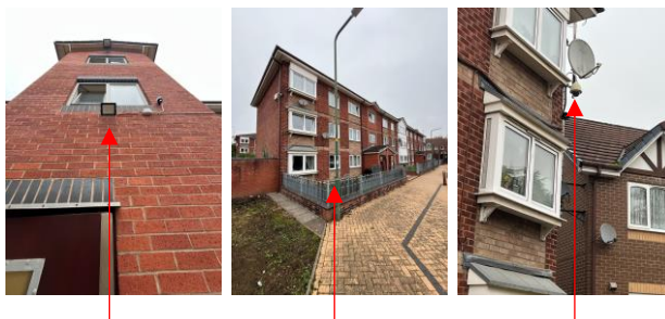
Rear lighting, Street lighting & CCTV
