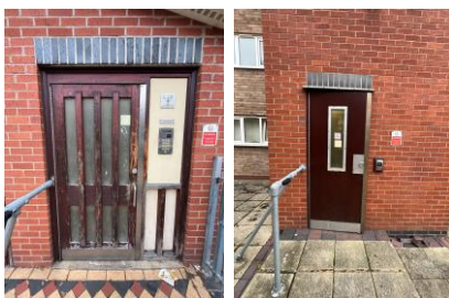
Front and rear entrances to block.
