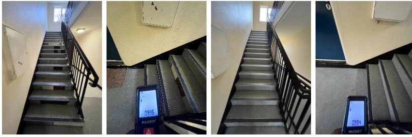
Ground to 1 st & 2 nd floor staircase.
