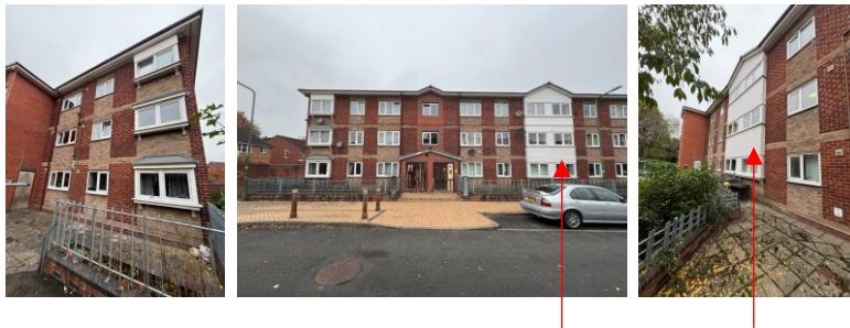
UPVC window units and UPVC Shiplap cladding to the front and rear
