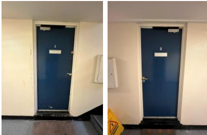
Ground floor flats 1,2,
