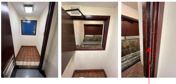
Bin store enclosure and smoke seals
