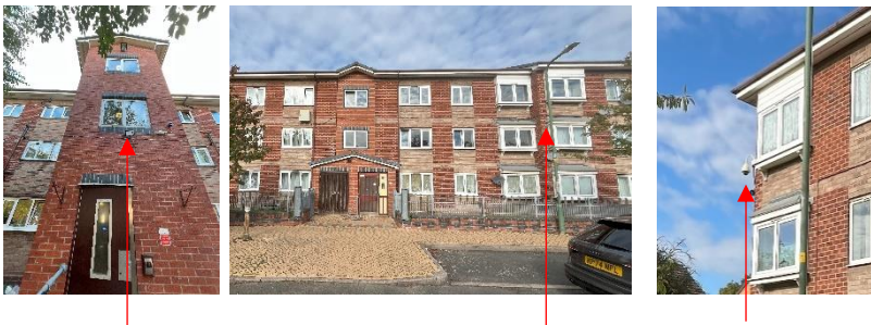
Rear external lighting, Street lighting & CCTV
