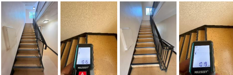
Ground to 1 st & 2 nd floor staircase.
