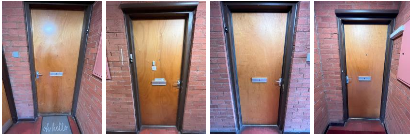
Ground floor flats 1,2,3,4
