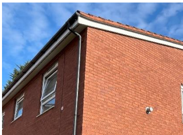
UPVC Facias boards with concrete roof tiles
