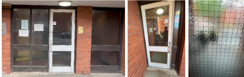
Timber constructed door entrance and Georgian Wired Glass
