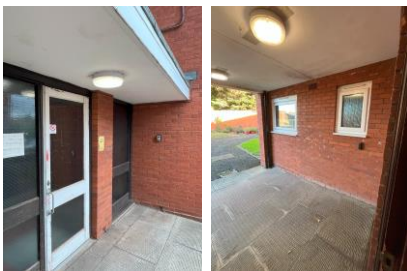
Front External lighting
