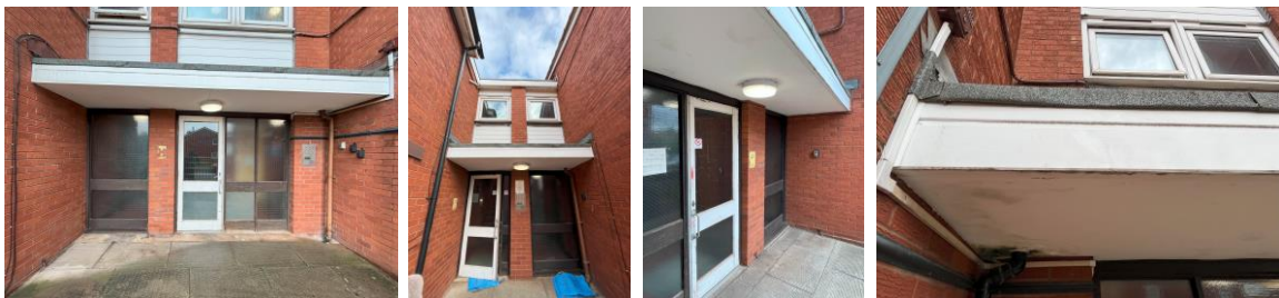
Canopies over front and rear entrances to both blocks.
