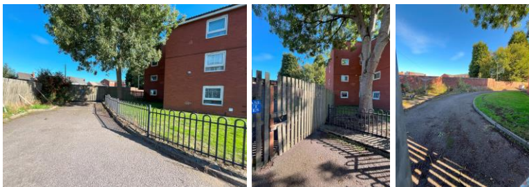
Metal railing and timber fencing to the courtyard at the rear.
