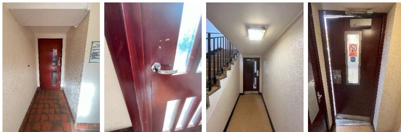
Communal doors before front and rear final exits doors.
