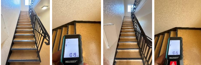
Ground to 1 st & 2 nd floor staircase.
