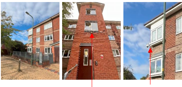
Street lighting, rear external lighting & CCTV
