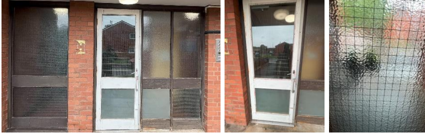
Timber constructed doors and Georgian wired glass
