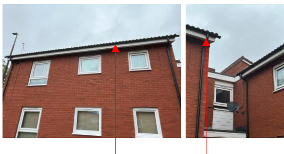
UPVC Fascias boards with concrete roof tiles.
