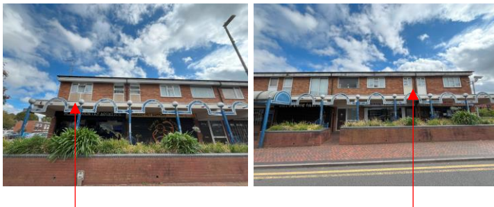
Spandrel panelling under the flat window units
