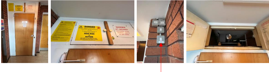
Lift, motor compartment and shaft access, shaft light and isolation switches.
