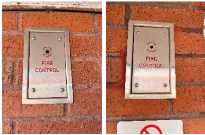
Front and rear firefighters Override Switch.
