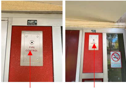
Block 1-6 & 7-12 Firefighters Override Switch.
