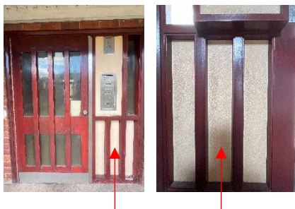
Spandrel panelling insets on the front entrance
