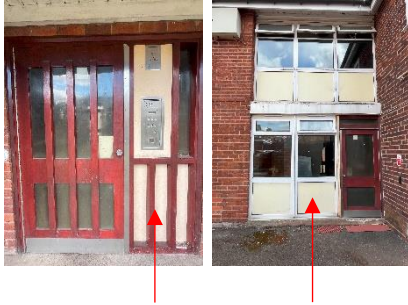
Spandrel panelling on the front and rear
