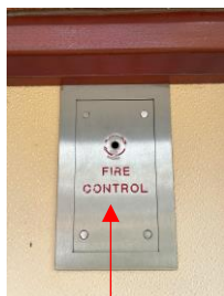
Firefighters Override Switch
