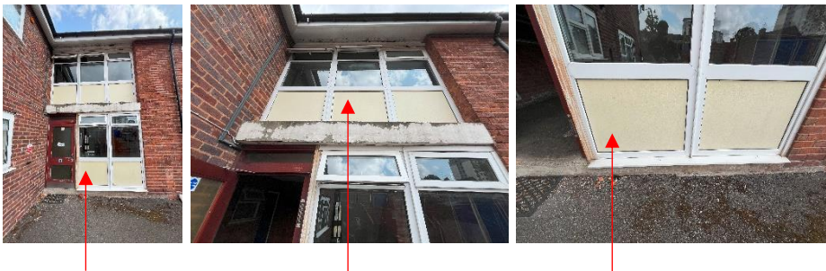
Rear Spandrel panelling under the window units
