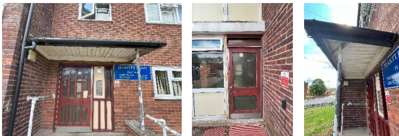
Front and rear timber constructed entrances and canopy
