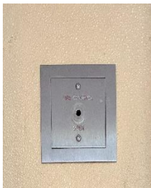
Firefighters Override Switch
