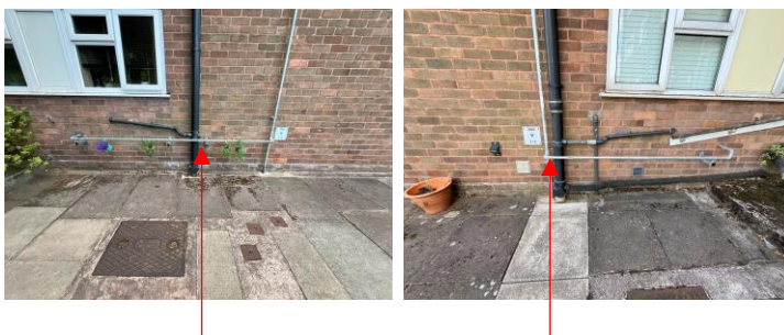
External gas pipework to the property
