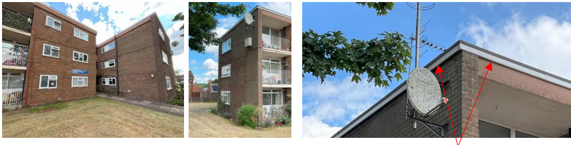
UPVC and felt roofline
