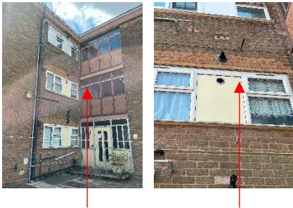
Extraction duct opening
