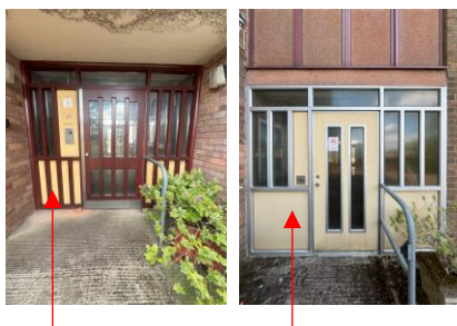
Spandrel panelling within inserts
