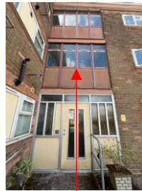
Front and rear Aluminium Framing
