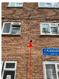
Exposed extarction ducting
