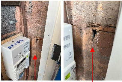
Cavity within brick work
