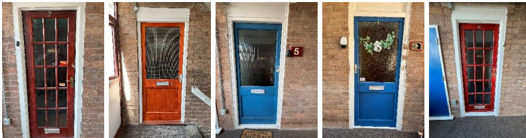
Flats 2,4,5,6,8 are non-Fire Rated doors with Yale and Mortice type locks
