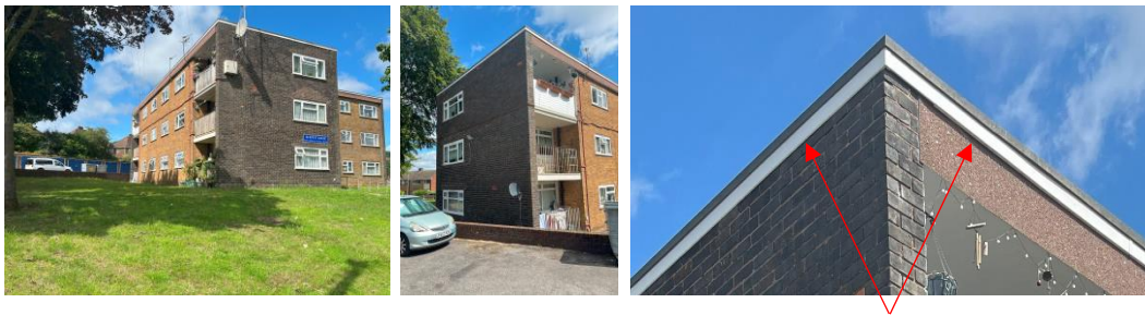
UPVC and felt roofline
