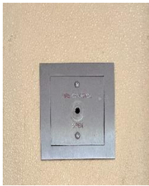
Firefighters Override Switch
