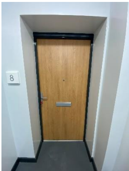
f) Flat 8 - Not reliably fully self-closing.
