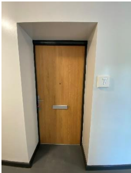
e) Flat 7 - Not reliably fully self-closing.
