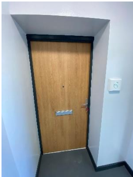
d) Flat 6 - Not reliably fully self-closing.
