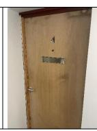
Section 7/23. Fire resistance of panel above door to water heater cupboard to be established (Flat 20 but generic statement). Upgrade to 30 minutes fire resistance if existing panel is inadequate.
