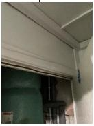
24) Flat 20 entrance door. The combined smoke strip to the frame on the slamming side of the door frame requires replacement.
