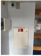
2) There is a dry riser that serves the building. The outlets are exposed and located on the communal lobby of each floor. Each exposed valve is secured with a cable tie. The caretakers check the cable tie is intact as part of their weekday inspections.
