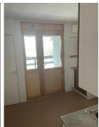
23) The panel above the fire door to the water heater cupboard does not appear to be fire resisting. The material should be confirmed and if required replaced with a 30-minute fire resisting board. This presents a low risk and can be incorporated within a future planned maintenance scheme.
