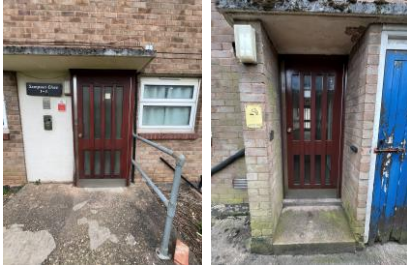
Front and rear entrances to block
