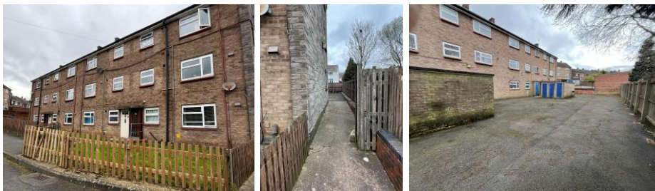
timber fencing perimeter and courtyard at the rear.
