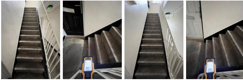
Ground to 1 st & 2 nd floor staircase.
