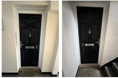
Ground floor flats 1,2
