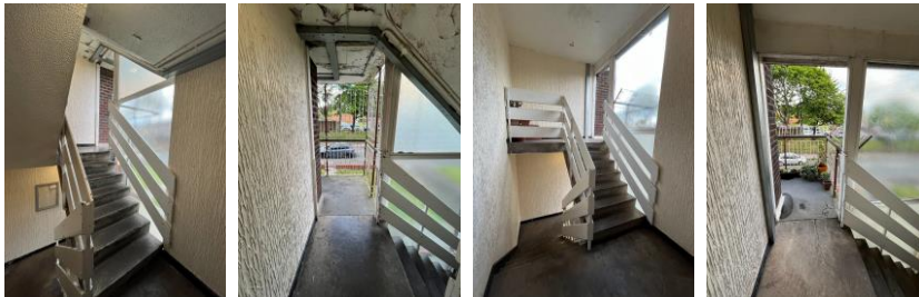
1st and 2 nd floor landing
