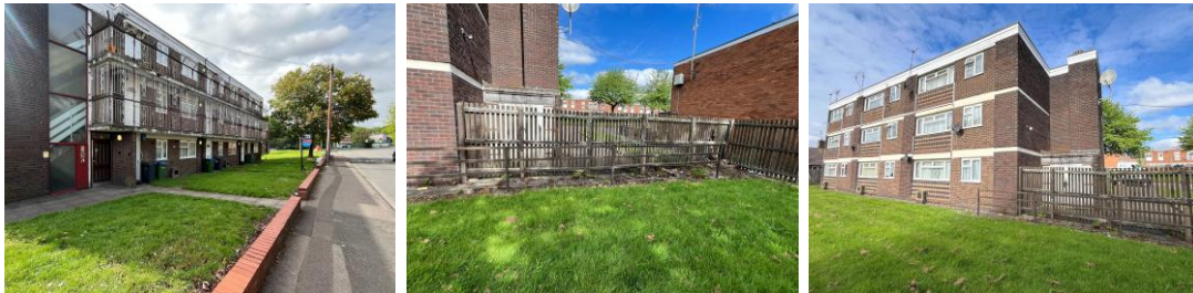
Brick and timber perimeter to the front and rear.
