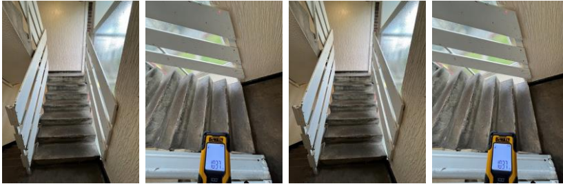
Ground to 1 st & 2 nd floor staircase.
