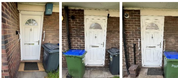
Ground floor flats 21,23,25
