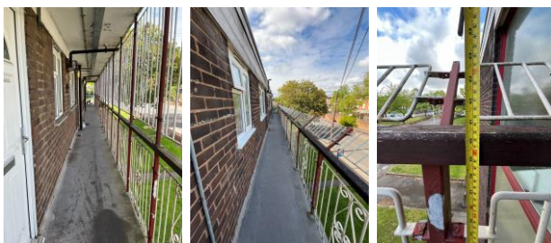
1 st & 2 nd floor open deck railings
