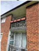
5) Timber soffits Noted. Email sent to repairs to advise of poor condition and to replace with non-combustible construction when works undertaken.
