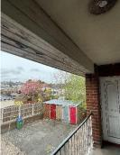
6) Plastic screen has been erected at ground floor. This prevents rapid dispersal of smoke which the open deck design provides. The screen is also combustible. The screen should therefore be removed. A drop of approx. 180mm will then be evident because a ramp has been built to access the flat entrance. Consideration should therefore be given to the provision of adequate guarding. Email sent to leaseholder management to pre warn residents.
