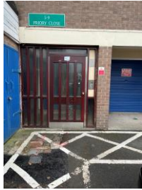
Front and rear entrances to block
