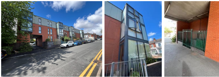
UPVC windows installed to flats and bin compound
