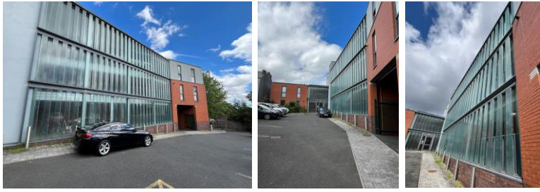
Rear elevation with staggered glass columns
