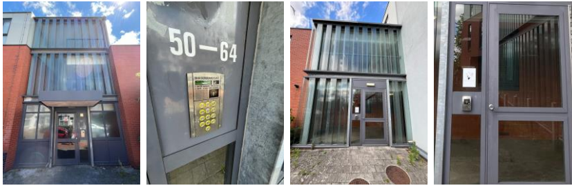
Door access control to the front and rear
