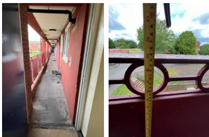
1 st floor open deck railings
