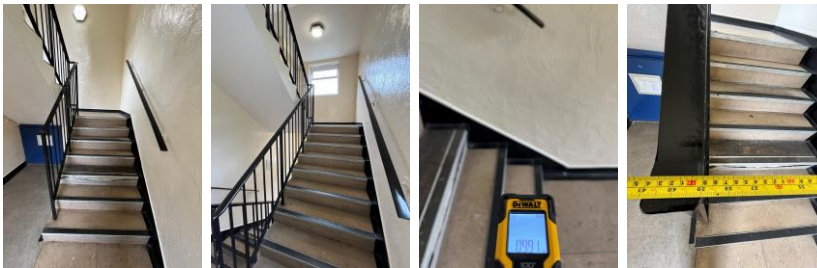
Ground to 1 st floor staircase.
