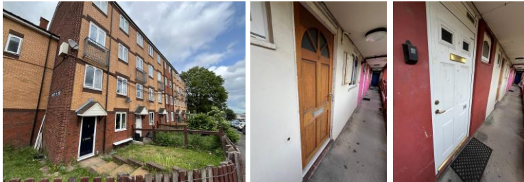
Ground & 1 st Floor flats entrance doors
