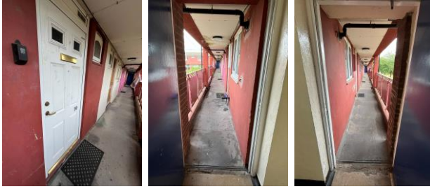
1 st floor flats 7-12
