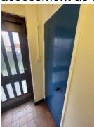
4) The final exit door is fitted with an automatic closing device and door entry system. This entry system is designed to fail safe i.e., door unlocked in the event of a power failure. This prevents residents being locked in or out of the building.
