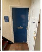
3) The only communal doors within the block are the final exit doors which are fitted with automatic closing devices that are checked on a regular basis by the Janitorial Teams as part of their daily checks. All blocks have a store door at ground floor level under the concrete stairs. These doors were not opened during the fire risk assessment as no key available.
