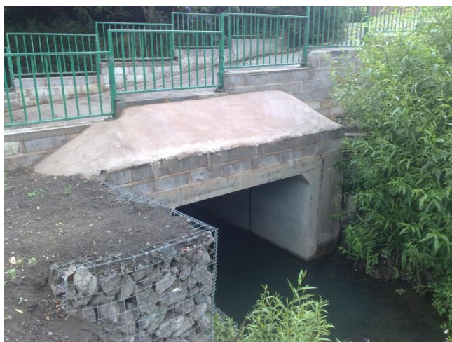
Figure 2 - Oversized culvert installed at Rushall Close, Wordsley in 2011
