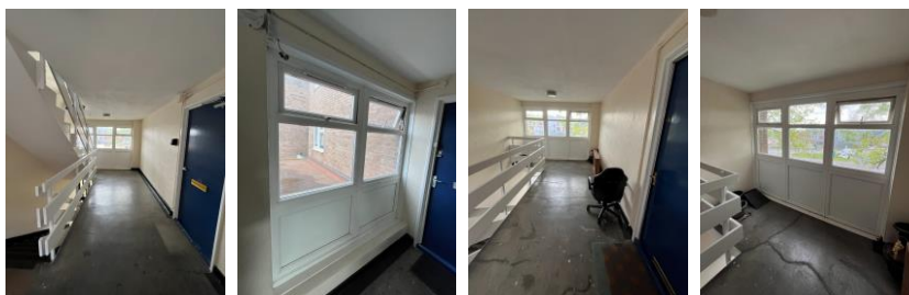
1st and 2 nd floor landing
