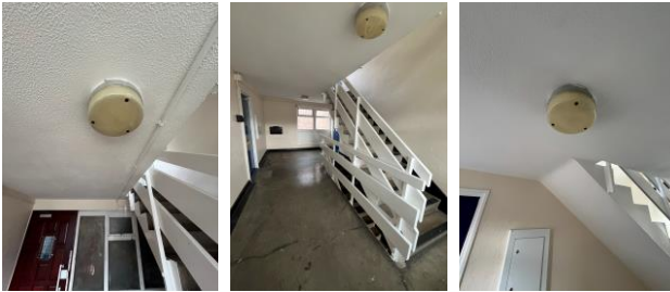
Communal corridors on ground, 1 st and 2 nd floors
