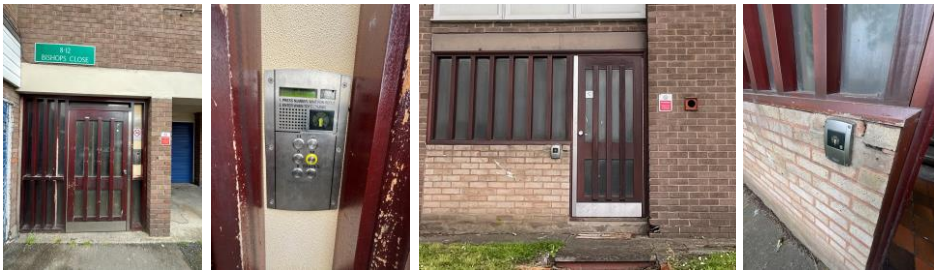
Front and rear entrance doors with access system.
