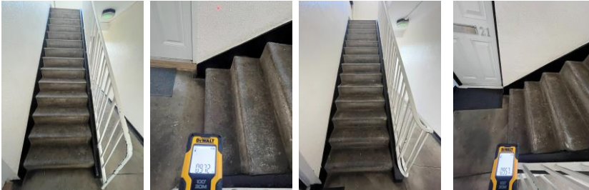
Ground to 1 st & 2 nd floor staircase.
