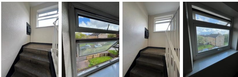
1 st and 2 nd floor landing
