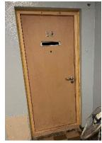
68) Floor 3. Staircase door not positively shutting into frame.
