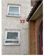
3. All communal windows to the protected staircase and single storey final exit are powder coated aluminium single glazed units.
