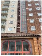
10. The ventilated block work to the chute rooms on the rear elevation have been externally covered with pest control netting. The netting will be permanently removed during significant refurbishments works that are anticipated to begin in the near future.
