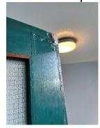
53) Floor 7. Staircase door frame. Stop to be re-nailed.
