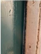
43) Floor 9. Staircase door not adequately shutting at time of inspection. Grit removed from under door. Issue resolved.
