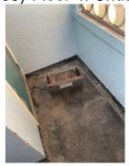
66) Floor 4. Chute room. Stop to fire door frame requires repair/replacement.
