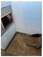
38) Floor 10. Staircase door not adequately shutting fully into frame.
