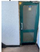
36) 11th Floor. Excessive gap between electrical cupboard doors.
