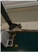
76) Floor 1. Staircase door. Stop to be re-nailed back to frame on leading edge.
