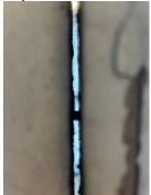
54) Floor 7. Corridor door into lift lobby not fully closing into frame.
