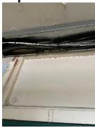
32) 12<sup>th</sup> Floor. Fire door separating corridor and lift lobby has no cold smoke strips top and side.
