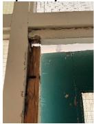
67) Floor 4. Door to flat 28. Does not positively shut and has no letterbox cover. (Pushchair removed at time of FRA)
