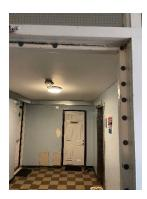
70) Floor 2. Staircase door not positively shutting.
