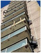
9. Ventilation panels to the front elevation consist of powder coated aluminium louvre vents.
