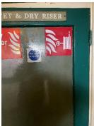
27) 13<sup>th</sup> Floor. Fire door to chute room. No cold smoke seal to top of door.
