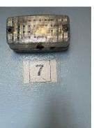
2) The centrally powered 24v units are provided to the communal landings, stairs and lift motor room. The batteries are located within the basement. Self -contained units are provided to the final exits, server and meeting rooms.
