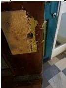
49) Floor 8. Chute Room. Fire door not adequately shutting.
