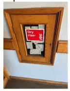
2) The dry riser outlets are located in cupboards adjacent the chute rooms at the lift end of the communal corridor on each floor. Each cupboard is secured with a budget lock. It was evident that telecommunication cabling within the riser cupboards does hang loose and is generally untidy. The cabling does not restrict the use of the riser outlets and will be made good as part of the significant building refurbishment works that are planned.
