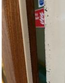
28) 12<sup>th</sup> Floor. Fire door separating lobby from corridor, by staircase, requires cold smoke seal on leading edge.
