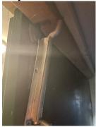
62) Floor 5. Corridor Fire door by dry riser requires repair as crack evident.
