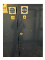
80) Ground Floor. Chute room. Door not positively closing fully into frame.
