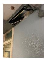
24) 13<sup>th</sup> floor. Fire Door, separating lobby from corridor, by electrical cupboard, does not shut as self-closer requires refixing.
