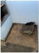
41) Floor 9. Cold smoke seal required to leading edge of staircase door.
