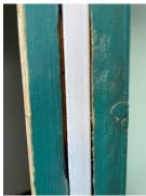
42) Floor 9. Door Frame to staircase. Door stop, to leading edge of door, to be re-nailed to enclose gaps.
