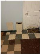
59) Floor 5. Staircase door is not positively closing fully into frame.
