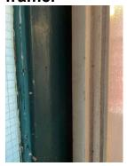
60) Floor 5. Corridor door into lobby, by staircase, has a damaged cold smoke seal.
