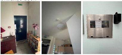
Based on the sample of properties accessed during the fire risk assessment the smoke alarms within resident's flats are installed to an LD3 and LD2 Standard (as confirmed by residents, no access gained).
