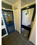
6) All communal doors are fitted with automatic closing devices that are checked on a regular basis by Caretaking Teams as part of their checks. Defective closing devices are replaced either by the Caretaking Team(s) or the in-house repairs team(s).
