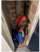
16) Service cupboard doors are Notional FD30S rated, secured with type 138 suited mortice locks. Residents have been provided with a key for access to their electricity meters.
