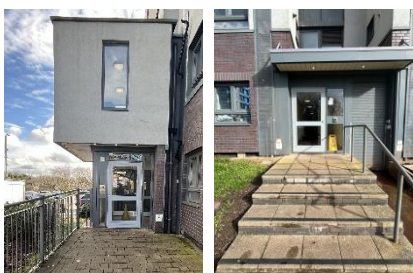
L/North Side R/South Side
