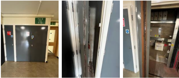
Dry Riser and electrical riser cupboards with nominal FD30 & FD60s doors
