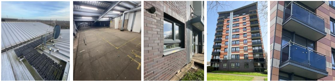
Steel framed roof, aluminium windows and cantilevered balconies
