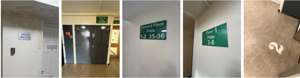
Floor signage in communal areas, adjacent to lifts and within staircas
