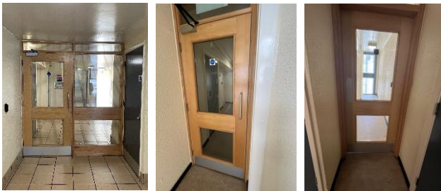
Ground, 5 th and 7 th floor communal lobby doors
