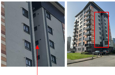
Kitchen windows near protective staircase
