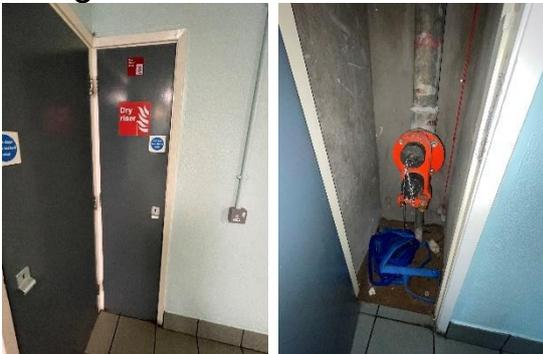
The dry riser outlet valves are located in cupboards on all floors directly above. These cupboards are also accessed utilising the 54 key from the firefighter's box.
