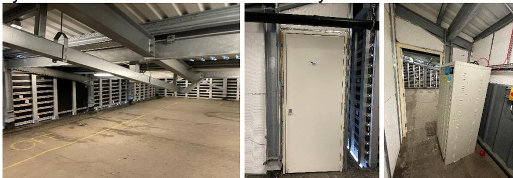
Automatic opening vents (AOV) have been installed in the stairwell between the 2/3, 4/5, 7/8 floors and also beside the chute room in all lift lobbies from the 1<sup>st</sup> to 8<sup>th</sup> floors.
