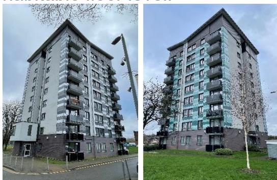
The typical structure is constructed as a reinforced concrete frame which was cast in-situ with an RC slab supported off cast in-situ RC walls/columns which stack vertically throughout. The concrete beams and columns are at regular centres and distributed evenly across the building. The typical floor slab is between 150-200mm thick.
