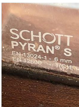
Etching to all glazed partitions / screening.
