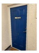
7) The corridors / staircases are protected by use of self-closing FD30s fire doors with combined intumescent strips / cold smoke seals and vision panels consisting of Georgian wired glazing.
