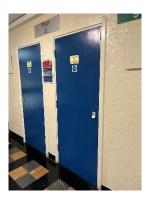
6) Individual flat doors are FD30s rated composite doors sets, the majority manufactured by Premdor doors, see section 7.
