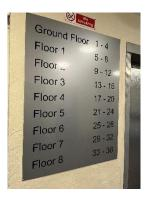
7) Photoluminescent wayfinding signage depicting floor level and flat numbers are fitted to the walls on all floors and to the wall of each landing on the communal staircase. Signage that meets the requirement of ADB and Fire Safety (England) Regulations 2022.
