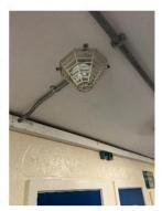
10) There are AOV vents on the 7<sup>th</sup>, 4<sup>th</sup> and 1<sup>st</sup> floors. The indicating control panel is sited in the main entrance foyer. The switch is operated by a key which can be found in the firefighter's white box.
