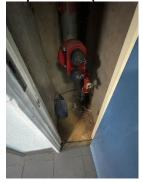
16) Service cupboard doors are FD30S rated, secured with type 138 suited mortice locks. Residents have been provided with a key for access to their electricity meters.
