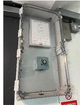
Dry riser outlets are in cupboards on all floors within the flat lobbies. The dry riser inlet is located in a cupboard in the ground floor lift lobby.
