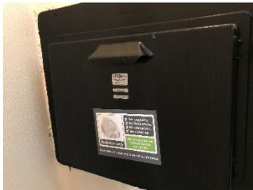
The bin chute leads to a bin store located on the ground floor accessed externally at the rear elevation of the block behind a roller shutter, the block is also taking part in a recycling project with the bins being stored at a safe distance away from the block.
