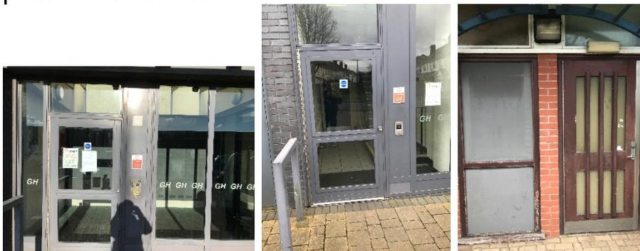
Front, side, and rear entrances utilise fob access in order to gain entry to the block with the front entrance also utilising a fire fighters override switch in the form of a drop latch system.
