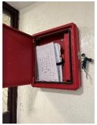
The dry riser inlet cupboard is in the ground floor lift lobby. Dry riser outlets are available on each floor lobby  $(1^{st} - 8^{th})$
