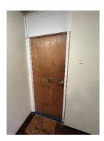
c) Flat 26 - Flat entrance door has excessive perimeter gaps. There is a 6mm latch-side gap and a 6mm head gap, requiring adjustment. See action 7/21c.
