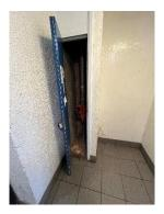
2) There is a dry riser outlet on each floor lift lobby, secured within a riser cupboard, the cupboards are locked with a suited key.
