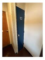
7) Individual flat doors are FD30s rated composite or timber doors sets, the majority manufactured by Jeld Wen doors, see section 7.
