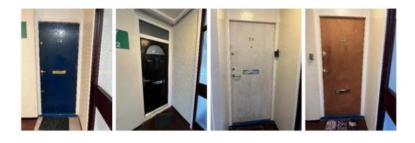
8) Void service cupboards were noted in the rear stairwell on floors 1, 4 & 7. All cupboards are secured with notional FD30s fire doors with combined intumescent strips and cold smoke seals, with suited mortice locks.
