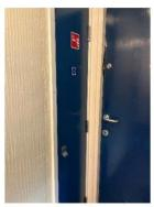
17) Service cupboards are 44mm notional fire doors with intumescent strips and cold smoke seals, secured with suited mortice locks to allow residents access to their electricity meters.
