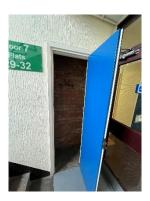
9) The lift motor room is secured with a 54mm notional FD60s door.
