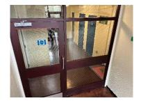
5) There's a nominal FD60s service cupboard door on each floor lobby, secured with a mortice type suited lock. The adjacent service cupboard is equipped with a nominal steel door with an internal fire-resistant board lining, minimum 30 minutes fire resistance. These doors are secured with a suited cylinder lock.
