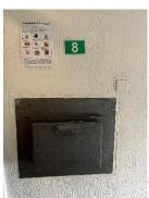
There are service cupboards on all floors with FD30s doors for electric meters and dry riser outlets, locked with a suited key.
