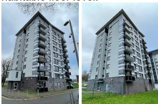
The typical structure is constructed as a reinforced concrete frame which was cast in-situ with an RC slab supported off cast in-situ RC walls/columns which stack vertically throughout. The concrete beams and columns are at regular centres and distributed evenly across the building. The typical floor slab is between 150-200mm thick.
