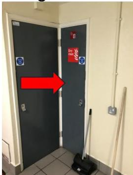
The dry riser outlet valves are located in cupboards on all floors directly above. These cupboards are also accessed utilising the 54 key from the firefighter's box.
