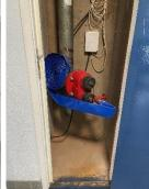
Dry riser outlets are available on each floor within the secured cupboards next to the lift car. Accessed is gained utilising the suited 54 key, also contained in the white box.
