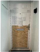
b) Flat 74 – Door is failing to fully self-close, adjustment to overhead self-closing device required.
