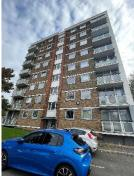
2) The side elevations were clad with a Wetherby mineral wool, silicon render system, fire classification A2 during a 2009 refurbishment. It was noted that a section of the render to the south facing side elevation of approximately 4m2 has come away exposing the mineral wool insulation beneath. The area has been cordoned off and the risk to fire remains low.
