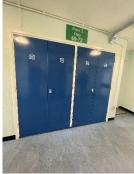
12) Dry riser inlet / outlets on lobbies are housed in cupboards with 44mm nominal fire doors with intumescent strips and cold smoke seals, locked with suited 54 key mortice locks. All outlet valves are secured in the closed position by cable tie.
