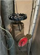
Automatic opening vents are installed to the 7<sup>th</sup> floor rear staircase. The override switch is on the 7<sup>th</sup> floor landing wall. Key is in the firefighter's white box.
