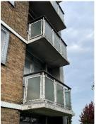
4) Communal windows are single glazed units housed in powder coated aluminium frames. Flat windows are double glazed units housed in timber frames with an external powder coated aluminium face.
