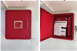
The bin store is protected by an automatic fire suppression system (drencher). The system is actuated upon the detection of smoke. The status panel for the system is located in the ground floor right hand service cupboard opposite the lift. The red beacon above the bin store roller shutter will illuminate when the system has actuated. The bin store is accessed using a key stored in the firefighters white box.
