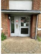
Both entrances have a door entry system with a fob reader installed. The front entrance only, has a firefighter door override switch by use of a drop latch key.
