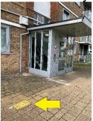
The dry riser inlet is next to the ground floor lift car. Accessed is gained utilising the suited 54 key, contained in the white box.
