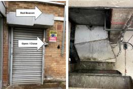
The bin chute is protected by an automatic closure plate. The system will operate following activation of the fusible link. The plate can be manually closed.
