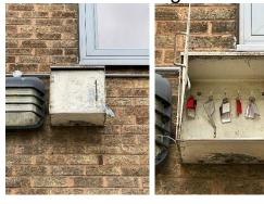
Access to the building is gained via the firefighter's door override switch utilising the drop latch key in the white box or alternatively the drop latch key stowed on the fire appliance.
