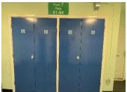
11) Dry riser inlet / outlets on lobbies are housed in cupboards with 44mm nominal fire doors with intumescent strips and cold smoke seals, locked with suited 54 key mortice locks. All outlet valves are secured in the closed position by cable tie.
