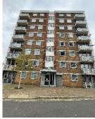
2) The side elevations were clad with a Wetherby mineral wool, silicon render system, fire classification A2 during a 2009 refurbishment.
