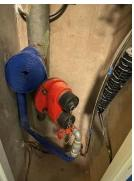
Dry riser outlets are available on each floor within the secured cupboards next to the lift car. Accessed is gained utilising the suited 54 key, also contained in the white box.
