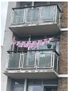
b) Flat 55 - timber screening installed to balcony unnecessarily increases the risk of potential external spread of flame.
