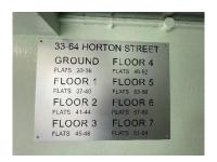
5) Photoluminescent wayfinding signage depicting floor level and flat numbers have been installed to the walls on all floors adjacent the lift car's and to the wall of each landing on the communal staircase. Signage that meets the requirement of ADB and Fire Safety (England) Regulations 2022
