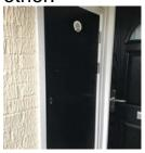
14) The store cupboard and meter / bin-store cupboards to either side of 1<sup>st</sup> floor flat front doors have non-fire rated timber doors.
