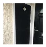
The store cupboard and meter / bin-store cupboards to either side of 1<sup>st</sup> floor flat front doors have non-fire rated timber doors.
