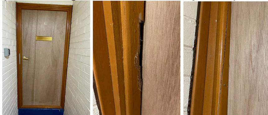
**B. Flat 8 has a temporary timber flush fire rated door.
