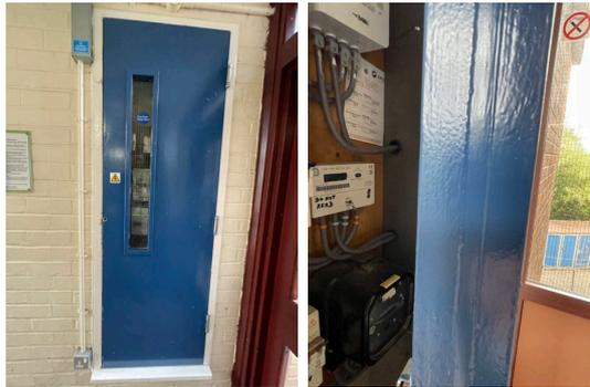
**B. Ground floor service cupboard has excessive gap on lock edge and is tight on hinge side.**
