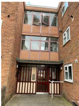
The block has a main entrance to the front elevation and a further exit located on the rear elevation. Front entrance has a door entry system with a fob reader installed and a firefighter override switch, the rear entrance has a fob reader.
