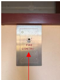
Firefighters Override Switch
