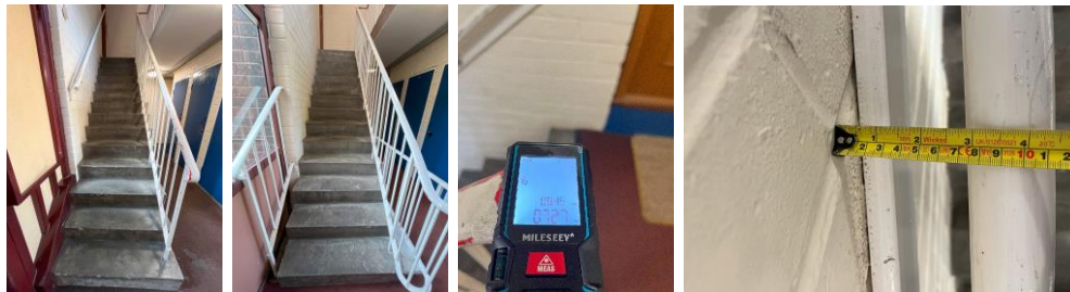
Ground to 1 st 1 st to 2 nd Ground floor rail comes out 110mm from the wall
