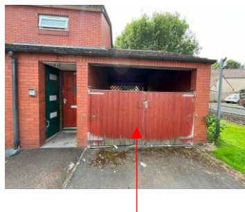
Car port compound
