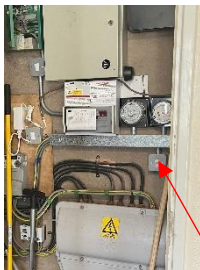
Emergency lights test switch
