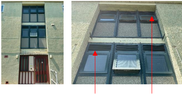
Louvered Venting above each window on the rear
