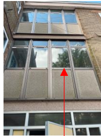
Front and rear Aluminium Framing
