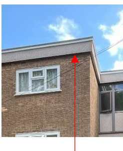
UPVC and felt roofing
