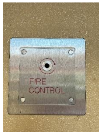
Firefighters Override Switch
