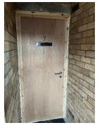
11) Accessed Flat 9 front door has a damaged door leaf. This door has no self-closing device and no combined intumescent and cold smoke strips. The glazing cannot be confirmed as being fire resistant. A replacement FD30s door set is required to be fitted. See action 7/11.
