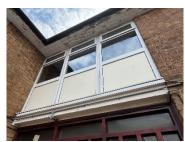
2) Individual flat windows are UPVC double glazed window frames. The windows in the communal staircases are UPVC window frames with openable vents. The communal staircase window frames are fitted with spandrel panels.
