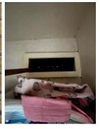
12) Flats 9 and 3 have UPVC windows fitted in the wall separating the flats from the common area. These window frames, including the glazing, do not appear to be fire-rated. Accessed flat 9's window was located in the bathroom. These non-fire rated windows should be replaced with a fire-resistant alternative during any future refurbishment of the block. See observations.
