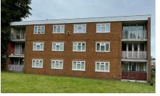
2) UPVC double glazed units have been installed to each flat and the communal stairwell.
